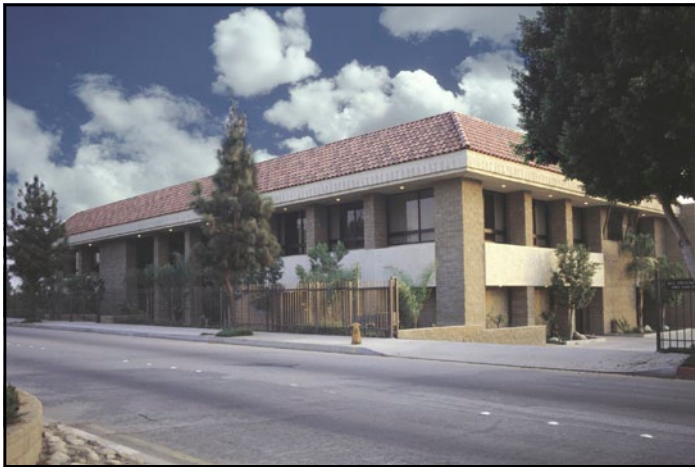
The Justice Brothers Museum is headquartered in this modern building along the old Route 66 in Duarte, CA. It's a super collection of automotive history and a great way to spend a few hours on the "Mother Road".
