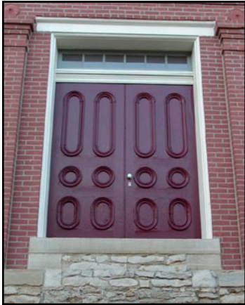
The fully restored Doors as they now appear.
